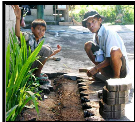
Paviours at children's home
